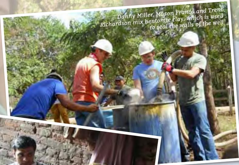
Danny Miller, Mason Franco and Trent Richardson mix bentonite clay, which is used to seal the walls of the well
